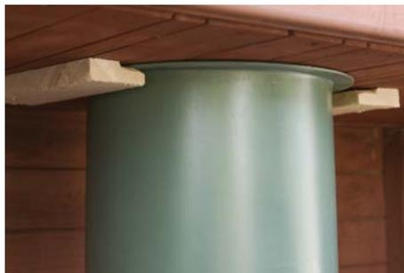
The ventilation pipe is preferably taken straight vertically alongside the wall. The ventilation pipe is equipped with a ventilation hat to prevent rain entering the pipeline. The place of the ventilation pipe can be adjusted with the flexible pipe. The Green Toilet package includes fixtures needed for the installation. The fixtures can be bended so that the pipes can be fastened with screws.
