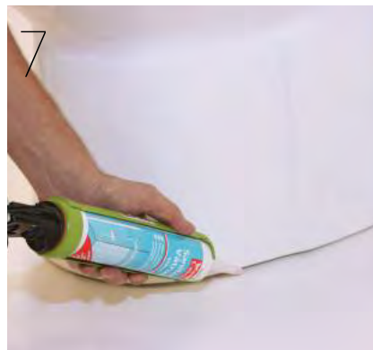
7 Glue the WC in place with transparent silicone. Limma fast WCn i golvet med transparent silicone.
